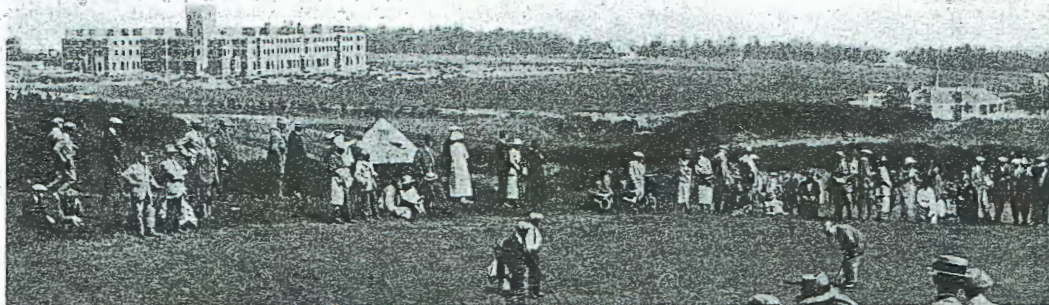
J.H. Taylor putting at "Denty Den," the 14th hole. The new hotel can be seen under construction.
